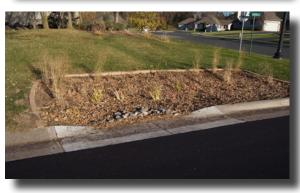
Rock inlet is cleaned and placed lower than curb-cut.
