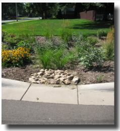
Pre-treatment features help reduce sediment load from clogging the bottom of the raingarden and buring plants. A clean inlet will help your raingarden to last longer.
