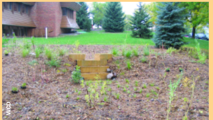
In fall 2007, one month after the project’s installation, the “spillway” connecting the two raingardens was still clearly visible.
