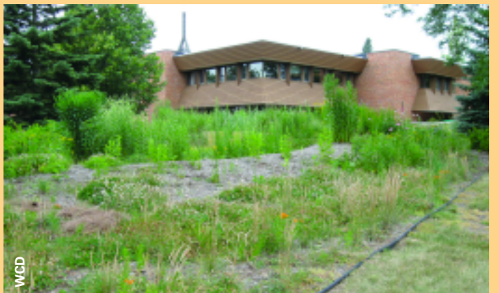
In summer 2009, nearly two years after installation, thick vegetation has covered the spillway and coneflower and butterfly weed can be seen in bloom.
