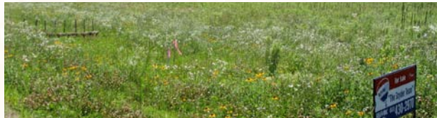
A combination of temporary and permanent erosion control measures, such as the hay bales and the permanent native vegetation planting seen above, reduce the overall site erosion potential. (SOURCE: WCD)
