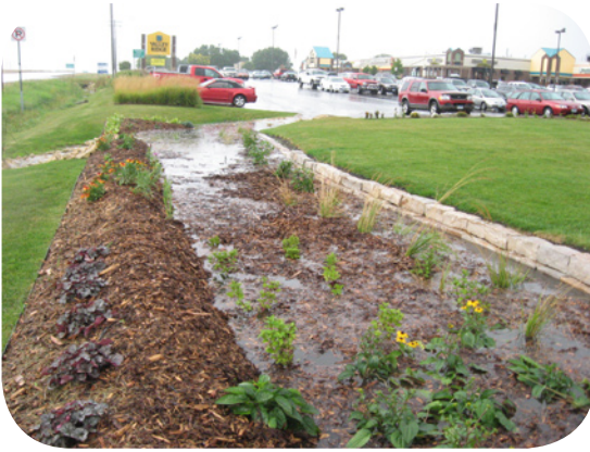
Above: The raingarden in front of Acapulco Restaurant one week after installation
